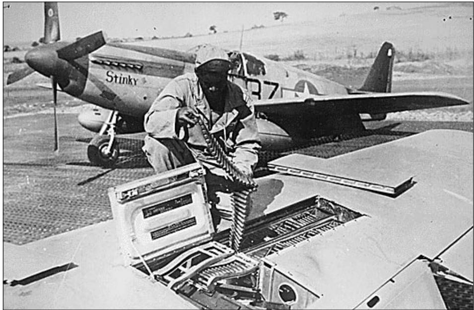
*An armorer of the 15th Air Force checks ammunition belts of the .50-caliber machine guns in the wings of a P-51 Mustang fighter plane before it leaves an Italian base for a mission against German military targets. The 15th Air Force was organized for long range assault missions and its fighters and bombers ranged over enemy targets in occupied and satellite nations, as well as Germany itself.*
